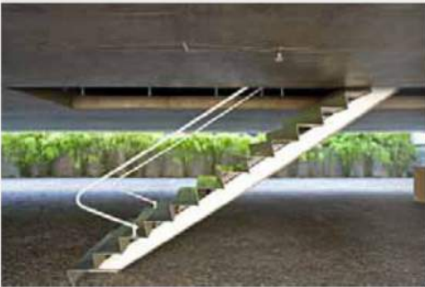
07812_060911_011D View of the elevating entrance staircase in down position
