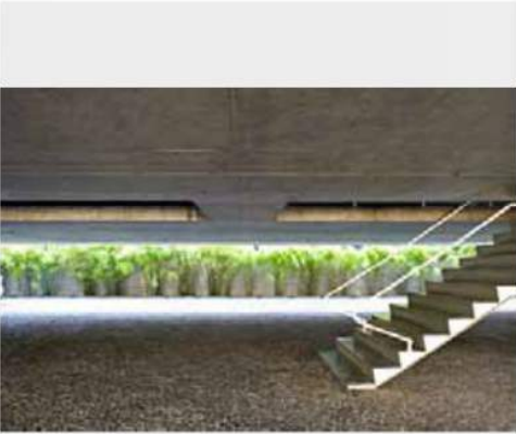
07812_060911_011D View of the elevating entrance staircase in down position
