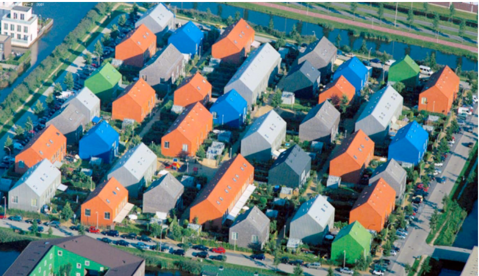
Fig. 2: Hageneiland housing , La Haye, 2001, source: mvrdiv.nl
