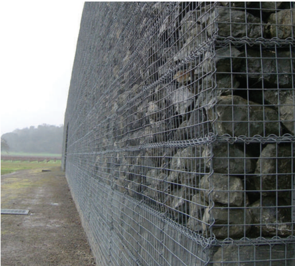
photo 16: Parement de gabions.
