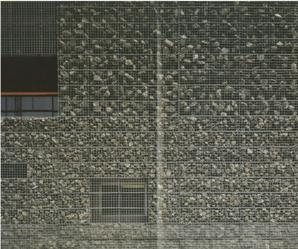
photo 15: Parement de gabions.
