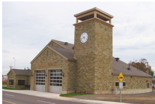
Figure 23 : La caserne de pompier de la rue Botsford (J.M. Giffin Engineering Inc., 2010, [En ligne], http://www.giffinengineering.com/botsford-st-fire-station/ )
